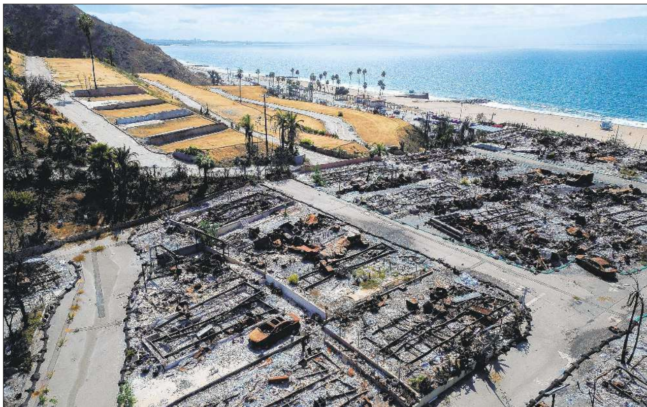
THE PACIFIC PALISADES Bowl Mobile Home Estates, unlike its neighbor, remains filled with fire debris.
